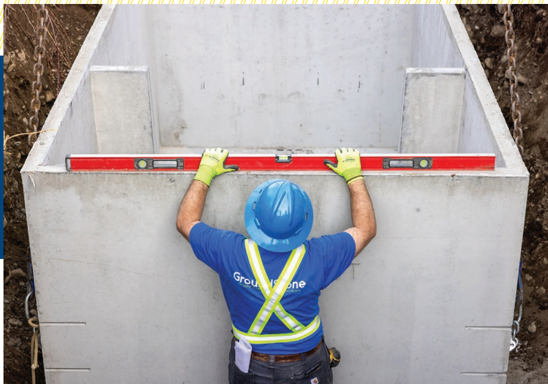
▲ Frederick checks a freshly placed concrete tank with a level while the chains are still attached in case adjustments need to be made.
