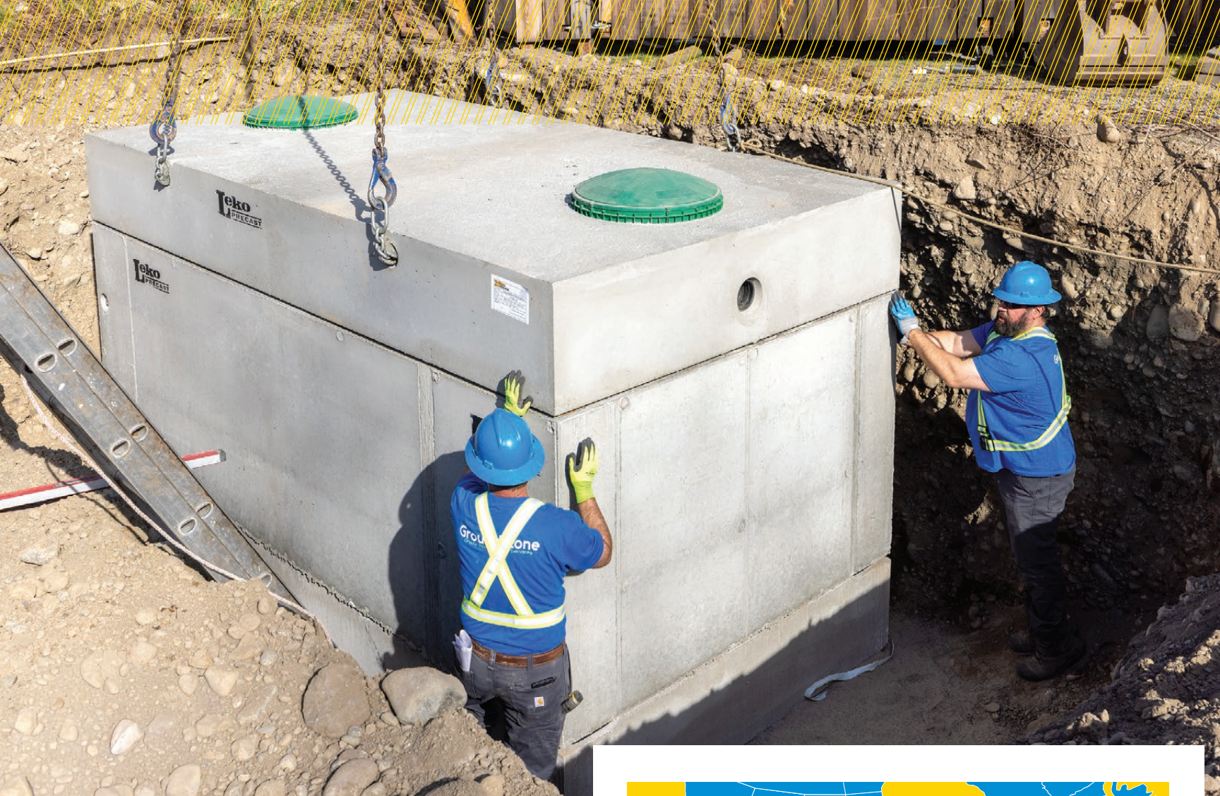
▲ Frederick (left) and Goncalves line up the lid of a Leko Precast 3,400-gallon tank as it's lowered into place.
